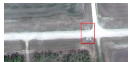
culvert pipes visible in Google Earth
